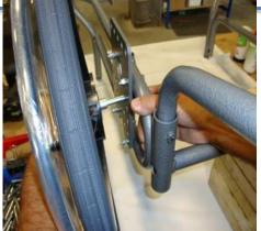
Insert a plastic anti-tip spacer ring into the open end of each caster post. Using the mallet, drive the Ring down as far as possible; then, using a slotted screw driver and hammer, drive the ring down further yet, until it fits snugly over the top of antitipper.
