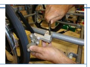
14 Test that the mag wheels and components have been installed correctly before use. Check that the mag wheels roll without obstruction when unlocked. Also check that the locks are close enough to bring the Mag Wheels to a halt when in "locked" mode.
